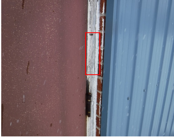
Photo 119: Photo of sample EXT-AS-06, Building Exterior, Wall – Caulking Around Door, 1.2% Chrysotile Asbestos.
