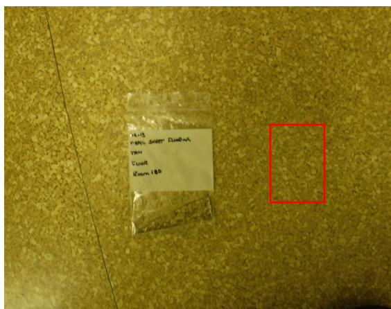
Photo 6: Photo of sample AS-13, Room 130, Floor – Tan Color Vinyl Sheet Flooring, 10.3% Chrysotile Asbestos.
