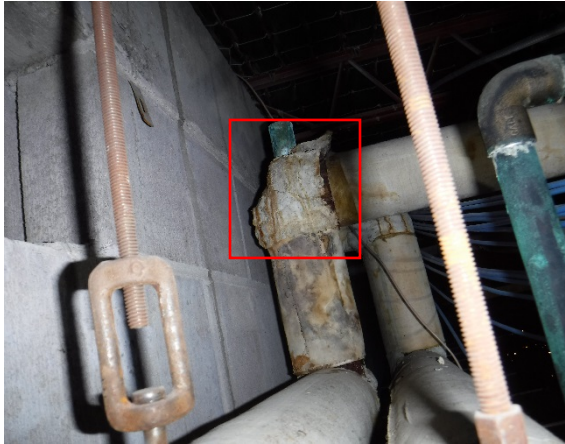
Photo 25: Example Photo of Poor Condition, Damaged ACM Piping Insulation, Fitting – Hallway (SW), Ceiling Cavity.
