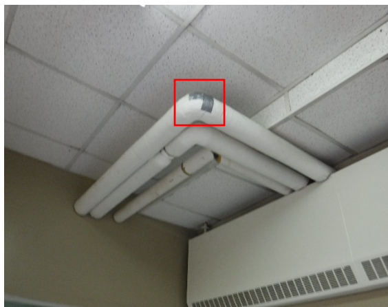
Photo 2: Photo of sample AS-08, Hallway (Main) – Piping Insulation, Fitting, 60% Chrysotile Asbestos.
