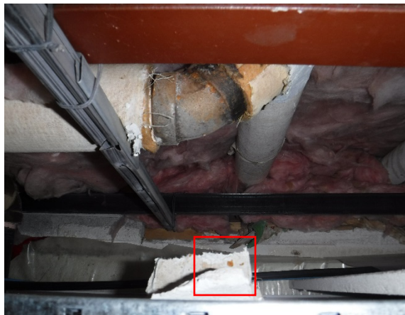
Photo 42: Photo of sample AS-26, Room 110 – Piping Insulation, Fitting, 55% Chrysotile Asbestos.
