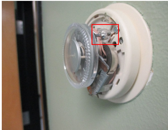
Photo 46: Example Photo of Mercury vial in older style thermostats observed throughout building.
