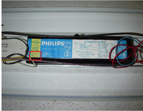
Photo 44: Example Photo of Inspected Lighting Ballasts – Men’s Washroom (SW), “Non-PCB”.
