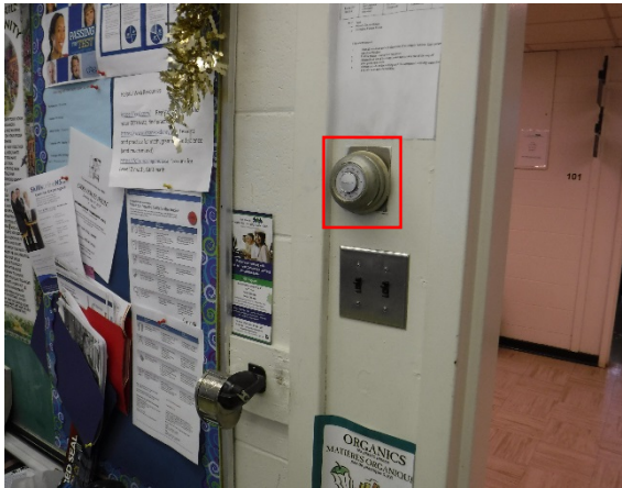
Photo 45: Example Photo of Mercury Thermostats observed throughout building.
