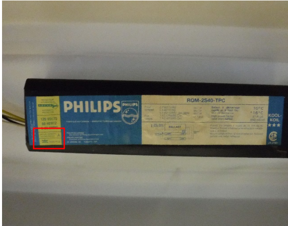
Photo 43: Example Photo of Inspected Lighting Ballasts – Hallway (Main), “Non-PCB”.
