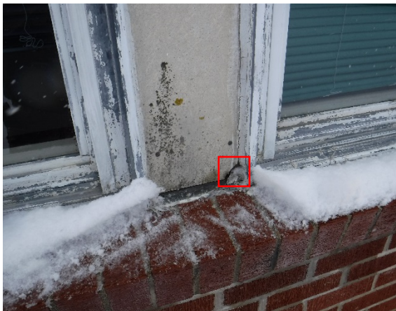
Photo 97: Photo of sample EXT-AS-02, Building Exterior – Caulking around Transite Panel, 2.2% Chrysotile Asbestos.
