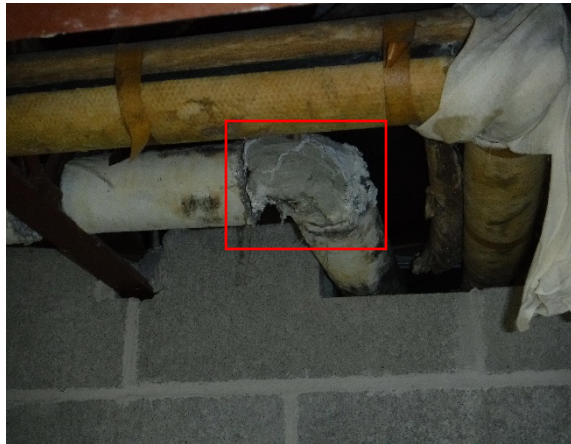
Photo 22: Example Photo of Poor Condition, Unwrapped ACM Piping Insulation, Fitting – Hallway (Main), Ceiling Cavity.
