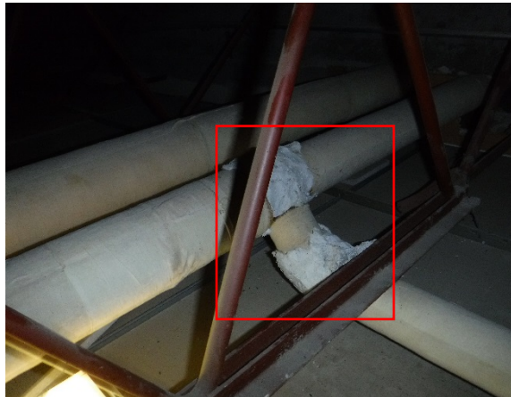
Photo 28: Example Photo of Poor Condition, Unwrapped ACM Piping Insulation, Fitting – Room 106, Ceiling Cavity.
