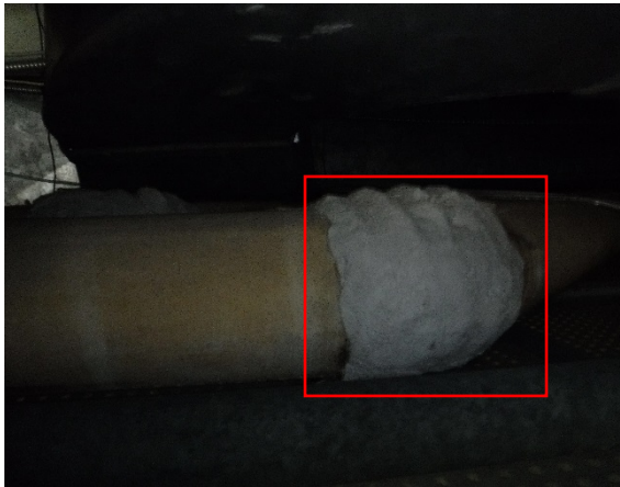
Photo 21: Example Photo of Poor Condition, Unwrapped ACM Piping Insulation, Fitting – Hallway (Main), Ceiling Cavity.
