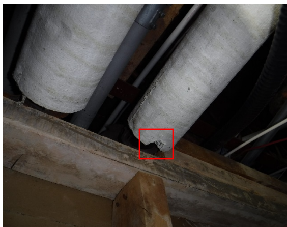
Photo 4: Photo of sample AS-11, Hallway (Main) – Piping Insulation, Straight Run, 60% Chrysotile Asbestos.
