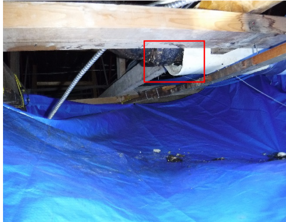
Photo 26: Example Photo of Poor Condition, ACM Piping Insulation damaged from Actively Leaking Pipe, Straight Run – Hallway (SW), Ceiling Cavity.
