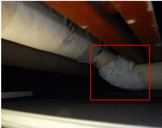
Photo 27: Example Photo of Poor Condition, Unwrapped ACM Piping Insulation, Fitting – Room 106, Ceiling Cavity.
