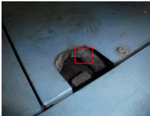
Photo 36: Example Photo of Non-Hazardous Fiberglass Insulation in Boilers – Mechanical Room.
